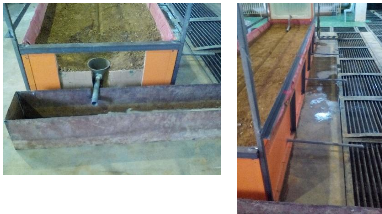
Figure 6: (a) Outlet (b) Groundwater flow using pipe UPVC
