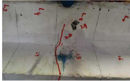
Figure 17: Top Front Cracking and Crushing at L5
