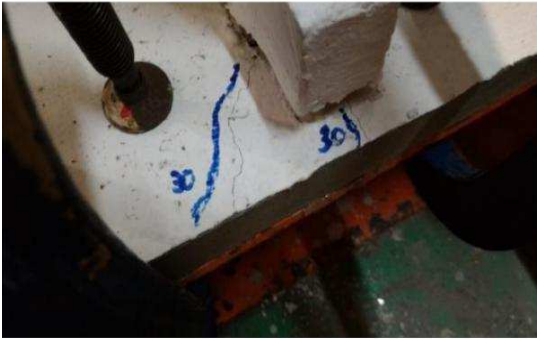
Figure 8: Crack at Top Side of Footing
