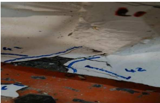
Figure 11: Spalling and Crushing at Footing
