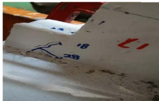
Figure 7: Crack Extended to Lower Part of Corbel
