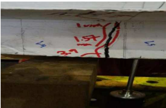
Figure 20: Crack Extended and Spalling
