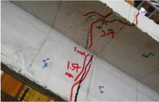
Figure 18: Back Bottom Cracking and Spalling at L4
