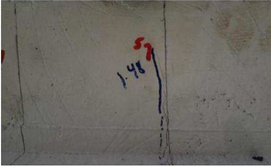
Figure 16: First Crack at 1.48 of Displacement
