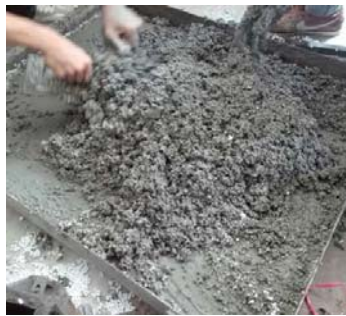
Figure 3: Mixing of Expanded Polystyrene with mortar.
