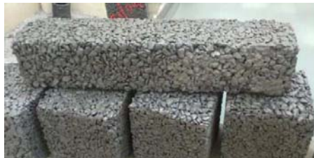
Figure 1: No-fines concrete used as pavement material [3].
