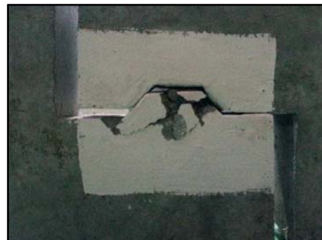
Figure 10: Crushing at key of Specimen C3
