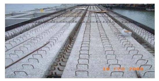
Figure 1.3: Shear Key in Precast Member
