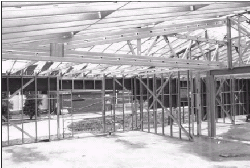
Figure 2.1 Cold-formed steel framing for residential houses [4]
