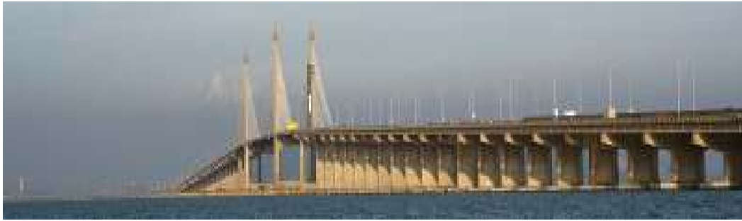
Figure 1.1: The Penang Bridge ( www.en.wikipedia.org ).
