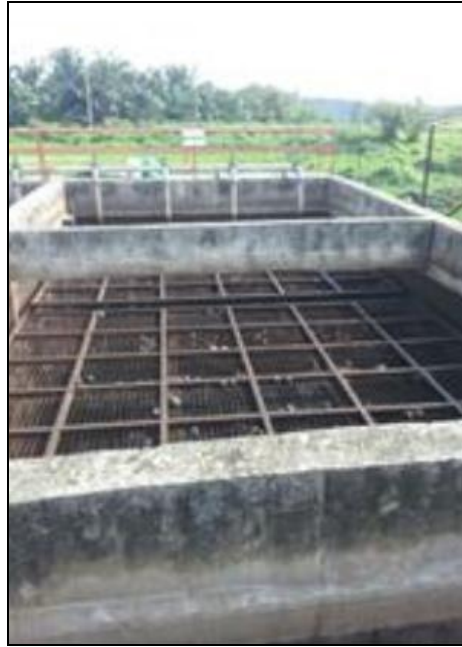
Figure 2: Mixed bed biofilm reactor during tank cleaning
