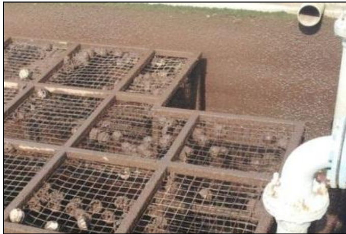
Figure 3: The reactor bed containing thousands of Biofilm Carriers
