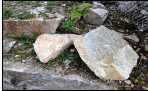
Figure 2: A boulder of rock fall
