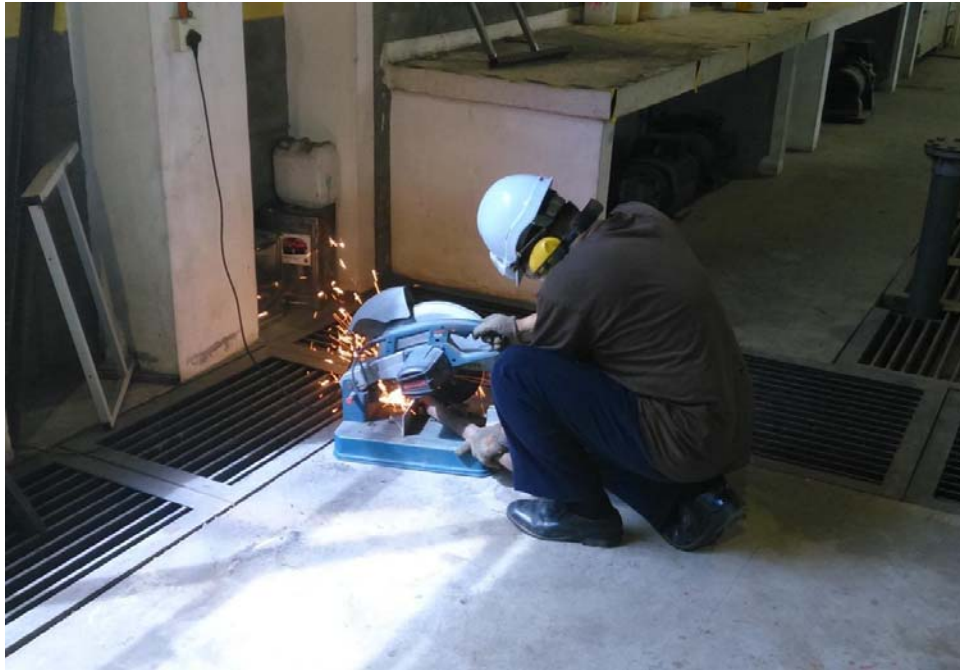
Figure 4: The steel was cut into several components
