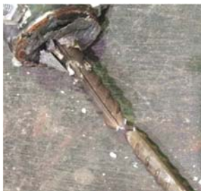
a) Bar Fractured
