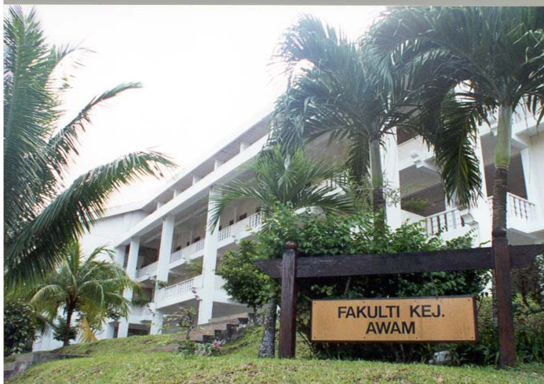
The Present Civil Engineering Faculty at Universiti Teknologi Malaysia, Skudai, Johor.
