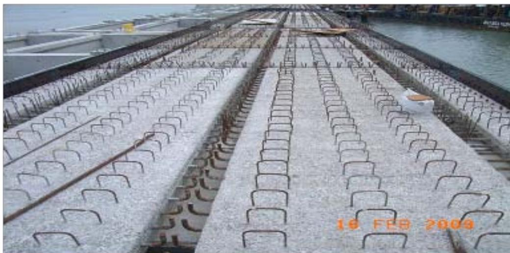
**Figure 1.3: Shear Key in Precast Member**
