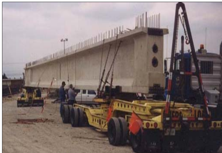
Figure 1.1: Length and weight limits on precast beams lead to splicing for longer spans
