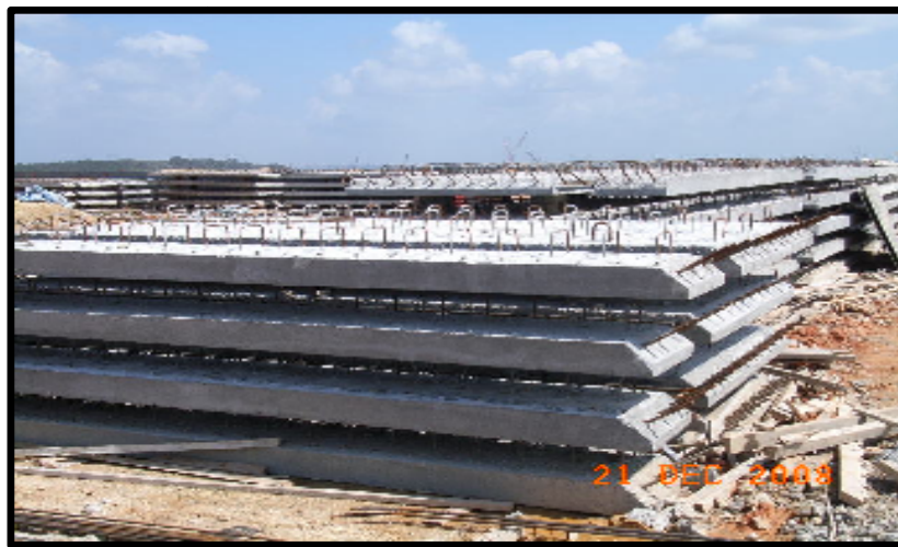
Figure 1.2: Precast Slab with Extruded Shear Key
