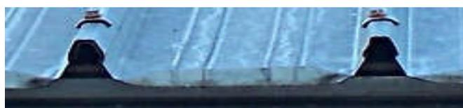
**Figure 2.5:** Klip-Lok Roof Sheeting.
