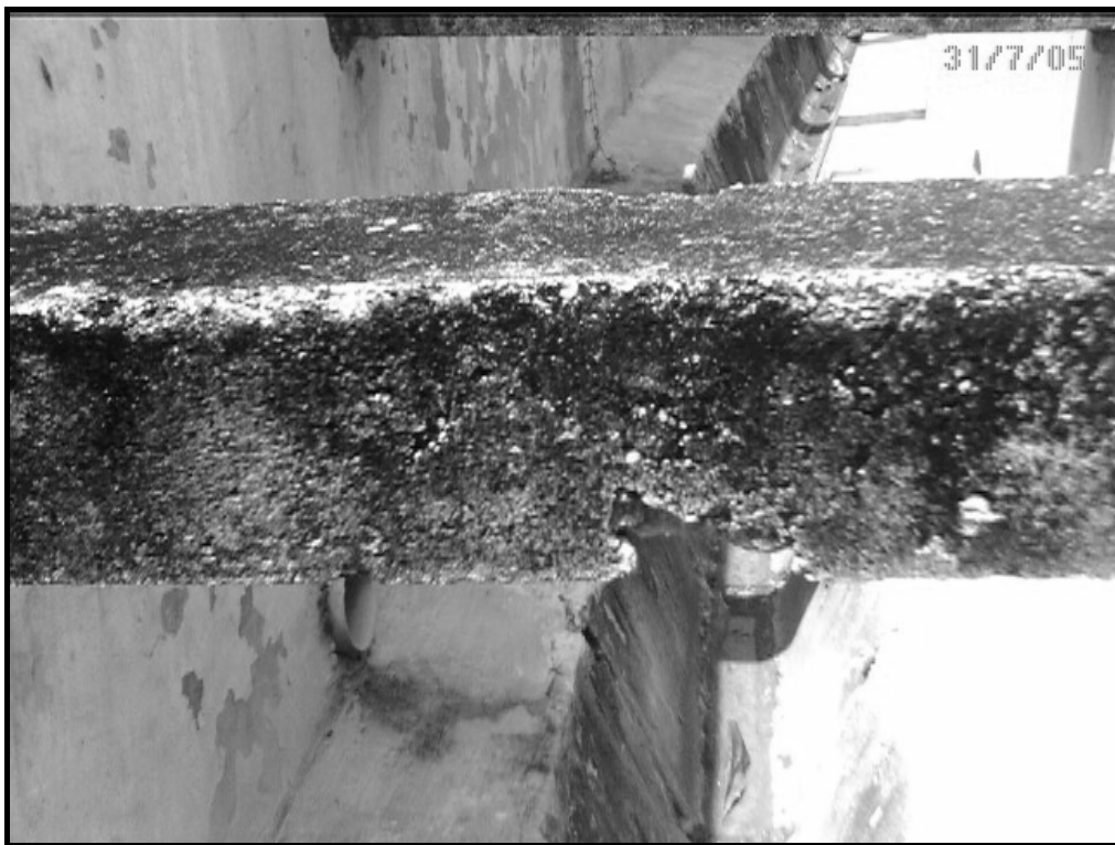
Figure 1.1: Figure depicts concrete have been severely eroded and start spalling.
