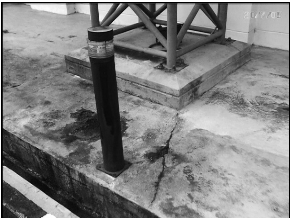
Figure 1.3: Figure depicts apron slab start cracking and surface is abraded.
