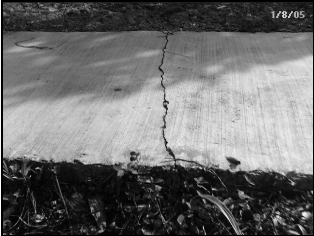
Figure 1.2: Figure depicts pathways slab transversely cracking.
